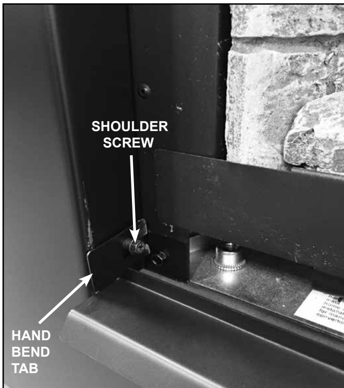
Figure 7 Hand Bend Tab & Shoulder Screw
